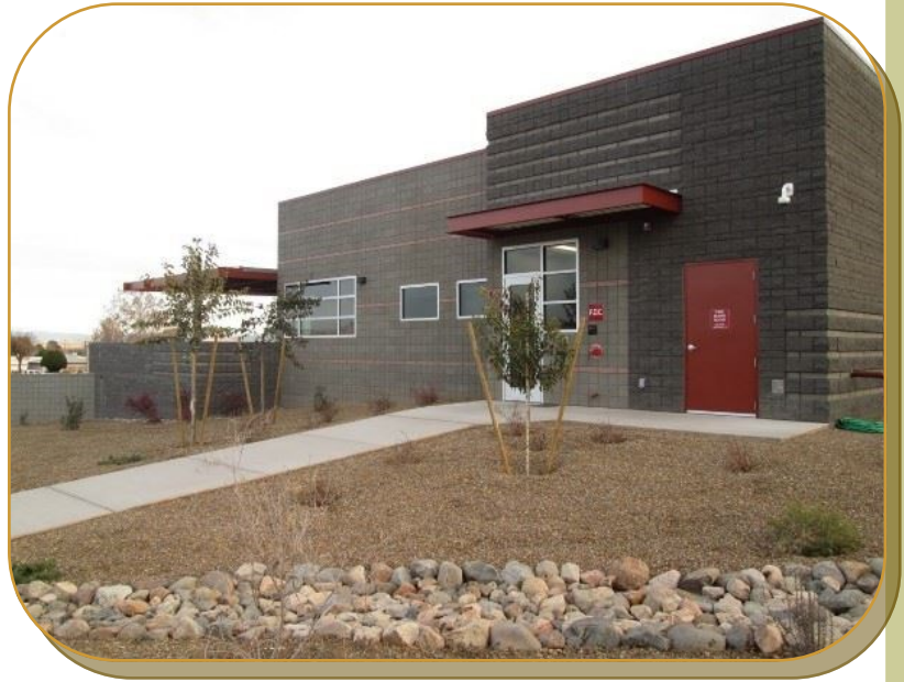
Cottonwood Public Safety Communications Center
