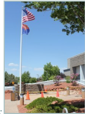
SFD Paver Project Under Construction — June 2012
