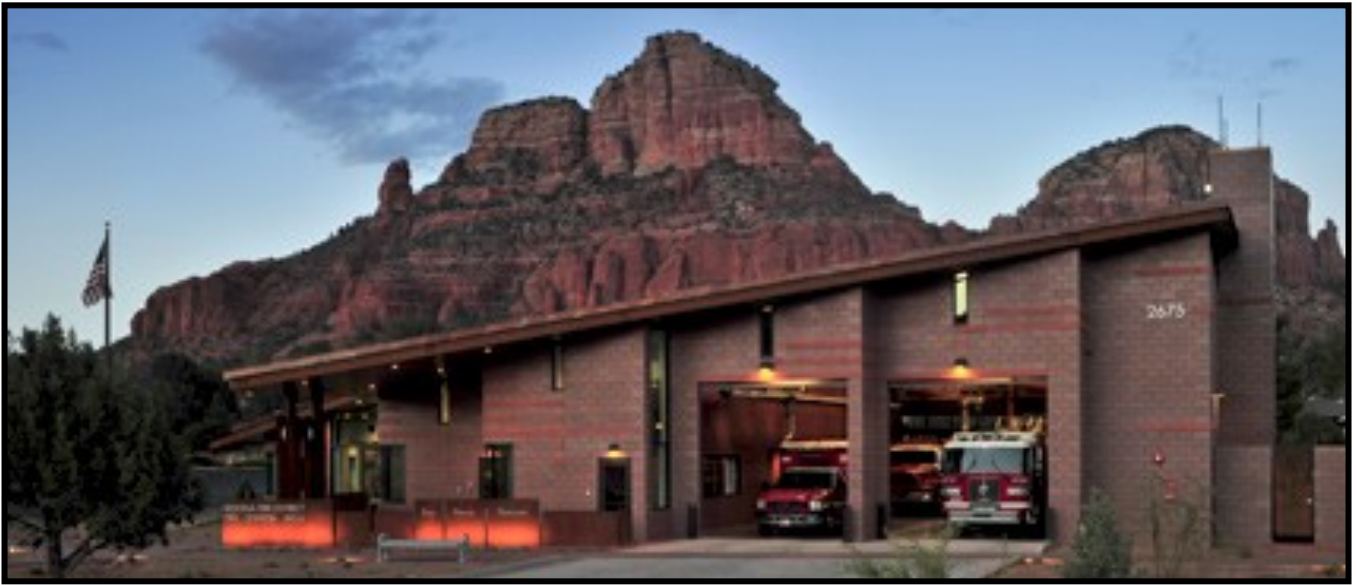
Station No. 6 2675 State Route 179 Built in 2014
