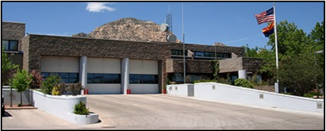
Station No. 1 2860 Southwest Dr. Built in 1990
